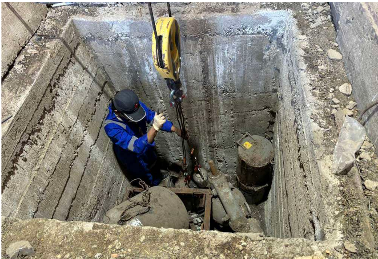
Recovery of devices containing ^{226}\text{Ra} sources from a subsurface storage facility in Mongolia.
