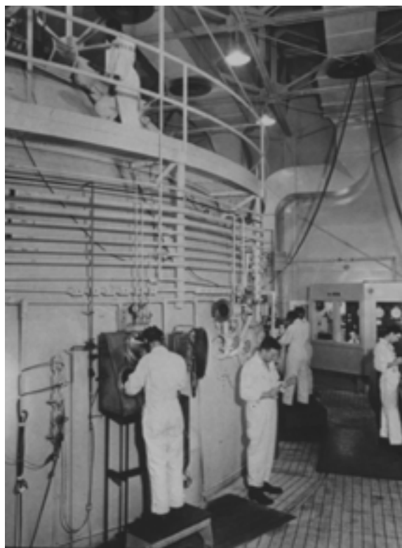
Fig. 19-1. These workers are standing outside the “8-Ball,” a 1-million-liter sphere used for testing static aerosols of biological agent preparations during the United States’s offensive biological warfare program. The building enclosing the 8-Ball and its supporting infrastructure were destroyed by fire in 1974. The sphere remains today as a historical monument at Fort Detrick, Frederick, Maryland. Photograph: Public Affairs Office, Fort Detrick, Frederick, Md. circa 1968.
