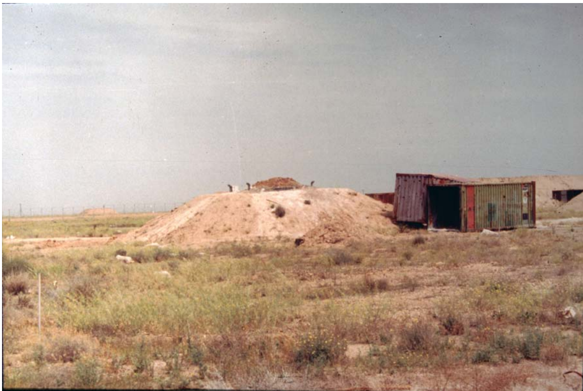
Figure III.XI.XVIII Semi-underground storage tank used for neutralization and entombment
