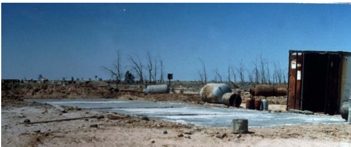
Figure III.XI.XX Thionyl chloride lagoon sealed with concrete after neutralization operations
