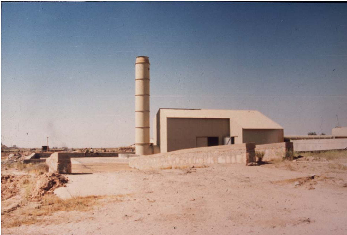
Figure III.XI.III Closer look at the furnace for the destruction of vapours from the hydrolysis plant (visible also on the left hand side of the previous photograph)
