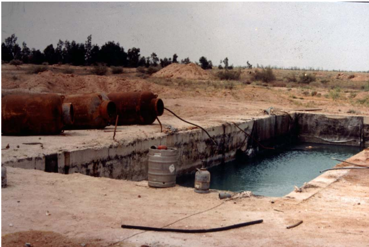
Figure III.XI.XX Thionyl chloride lagoon sealed with concrete after neutralization operations
