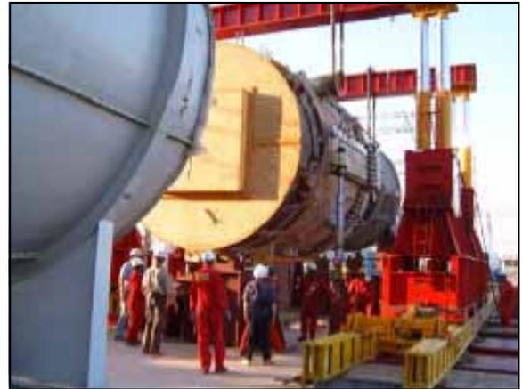
*The V-94 combustion gas turbine is being installed at a substation in Kirkuk; combined with a V-64 unit, this will add 325 MW to the national electric grid.*
