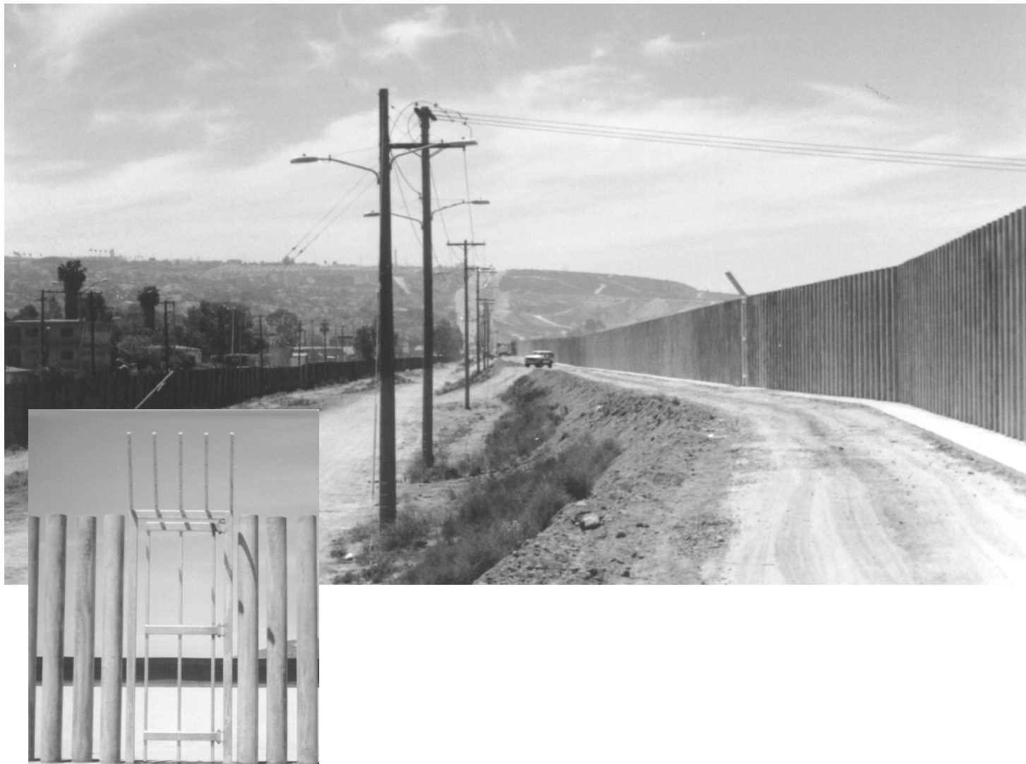
Figure 5: Bollard Fencing Being Constructed in San Diego, California
