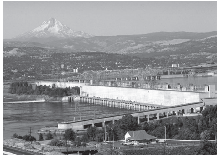
Source: DOD. Hydroelectric dam.
