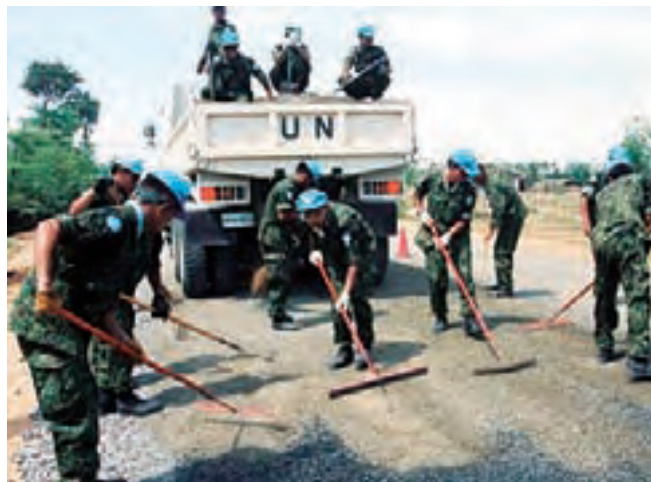
GSDF engineering unit repairing a low-cost paved road in Cambodia (1993) GSDF engineering unit repaired a total of approximately 100km of roads and around 40 bridges.
