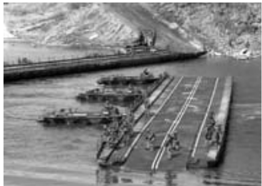
U.S. Army Corps of Engineers building a floating bridge across a river during a U.S.-ROK joint military exercise [AFP/JIJI]
