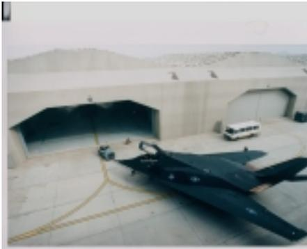
**Hardened aircraft shelters provide passive force protection for vital Air Force resources.**
