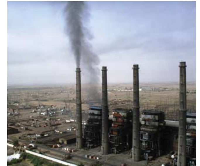
The Baiji Power Plant is a major producer of electricity for Iraq.
